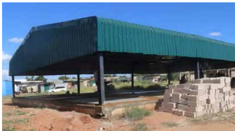
The new CDF Market Shelter under construction in Plan 2000 Township
